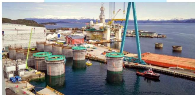
图7-2 干船坞注水浮起被湿拖设备
